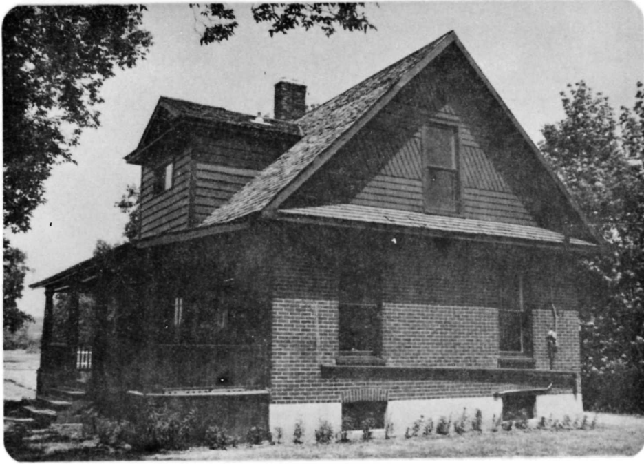
144 Lock No. 4, Batawa, July 1978. Dwelling House at lock built in 1924 and presently being used as lock office. 1
