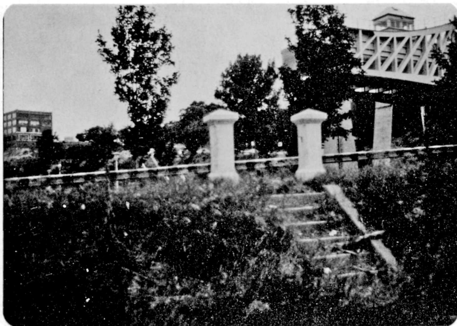
26 Lock No. 21, Lift Lock, Peterborough, August 1978. Pillars and staircase leading to dwelling house pathway south-east of lift lock. House was removed in early 1960's and only foundations remain. 1
