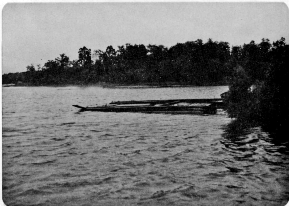
80 Near Lock No. 35, Rosedale, August 1978. One of old lock gates from wooden lock built in 1873 on Gull River near Rosedale and abandoned in 1910. Gate is presently being used as a wharf by Arkadia Trailer Camp.
