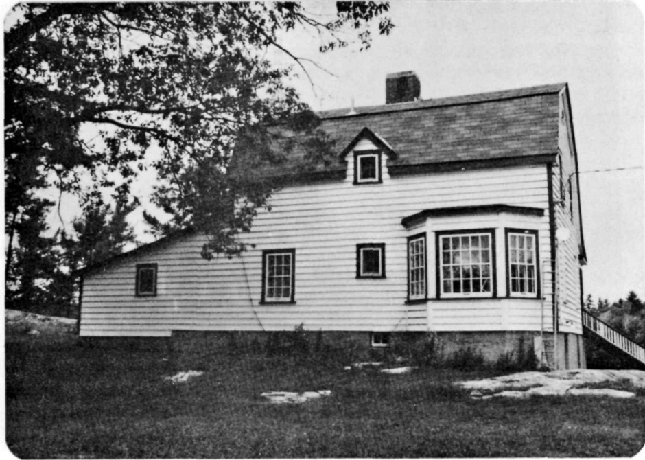
180 Lock No. 43, Swift Rapids, June 1978. Orillia Water, Light and Power Commission's dwelling house for power plant superintendent. Built ca. 1916 and still in use in its original location on the south side of the river at Swift Rapids (rear view).
